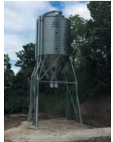
Silo on its own gantry
