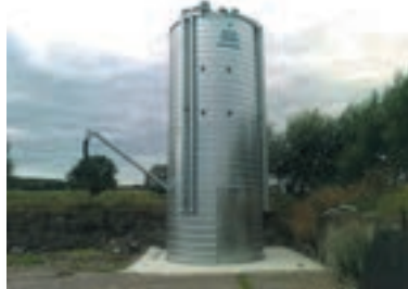
Enclosed Silo and Reverse Drive Auger
